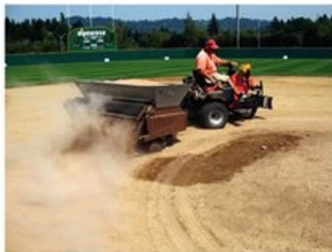
The Turfco tow-behind topdresser was used to add the infield dirt.
