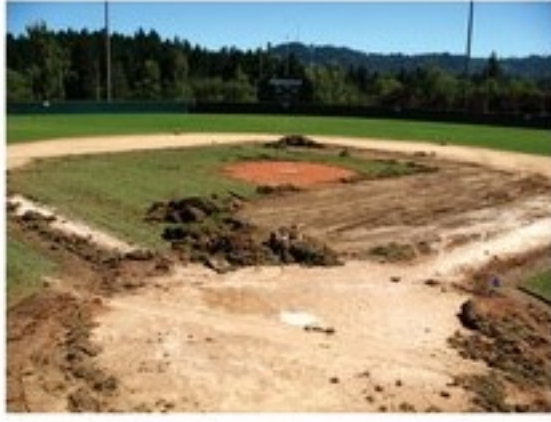
Turf removal worked from the base path toward the mound as the baseball field is converted for softball.
