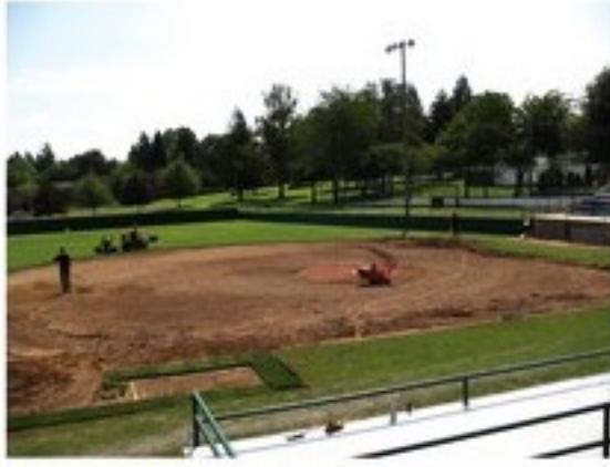
Most of the sod has been stripped and removed in preparation for the skinned infield for softball.
